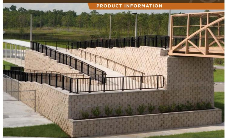
Designed for steep, sloping hillsides and other structural challenges, the Vertica® retaining wall system can be built to virtually any height in incredibly tight spaces – thanks to an impressive 2-degree batter, built-in lug locators, and a nearly vertical rise for less excavation and land loss. Typically used with geosynthetic reinforcement, Vertica blocks meet or exceed industry standards for strength and durability.
